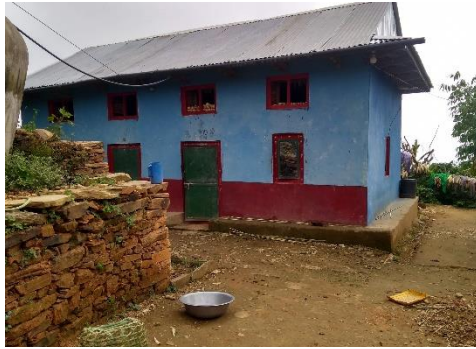
Photo 2: A typical house in Kavre
